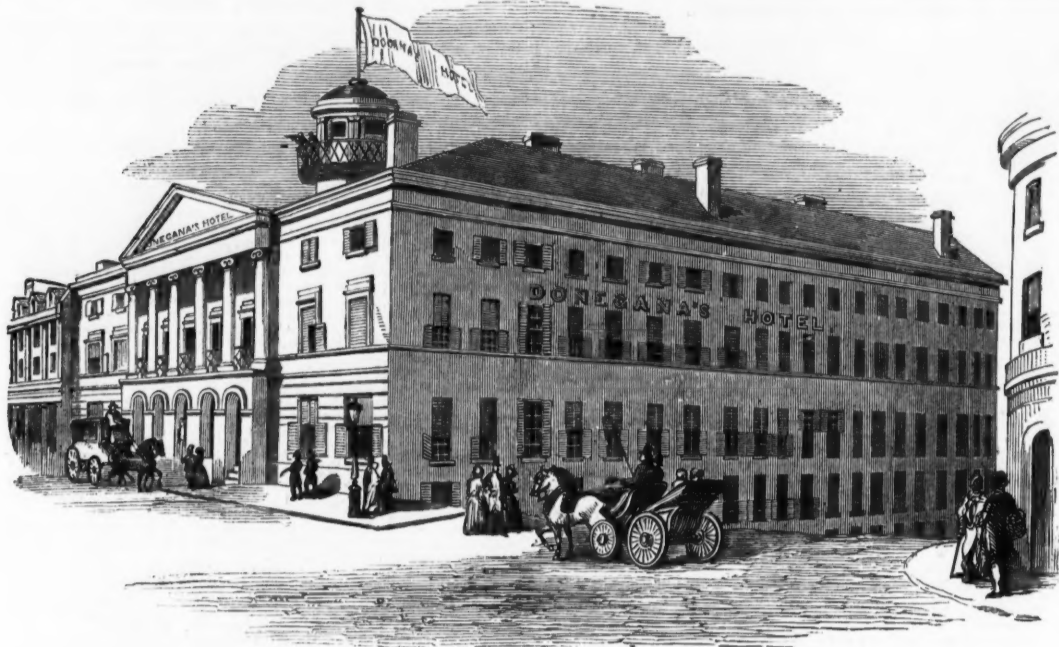
DONEGANA'S HOTEL, MONTREAL, DESTROYED BY FIRE ON AUGUST 16.
